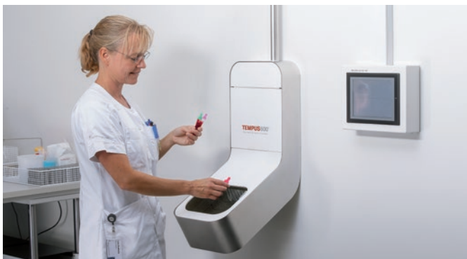
Samples arrive in the Receiving Tray where they are retrieved.
